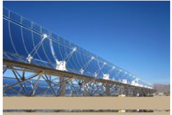
A demonstration system that features 16,579 square feet of 3M Solar Mirror Film 1100 and the Gossamer Space Frames to mount the lighter-weight mirrors at the Sunray Energy facility in Daggett, California, home of the longest operating parabolic trough solar facility in the United States.
