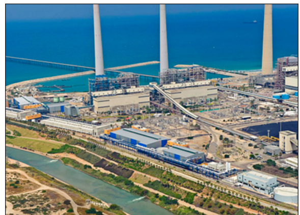
The desalination plant in Ras Al Khair, Saudi Arabia, produces more than a million cubic meters of fresh water a day.
