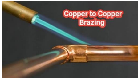
Copper to Copper Tube/Pipe Brazing
